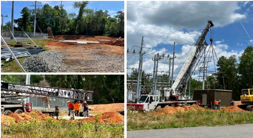
Placement of communication hut at the Stanardsville substation
