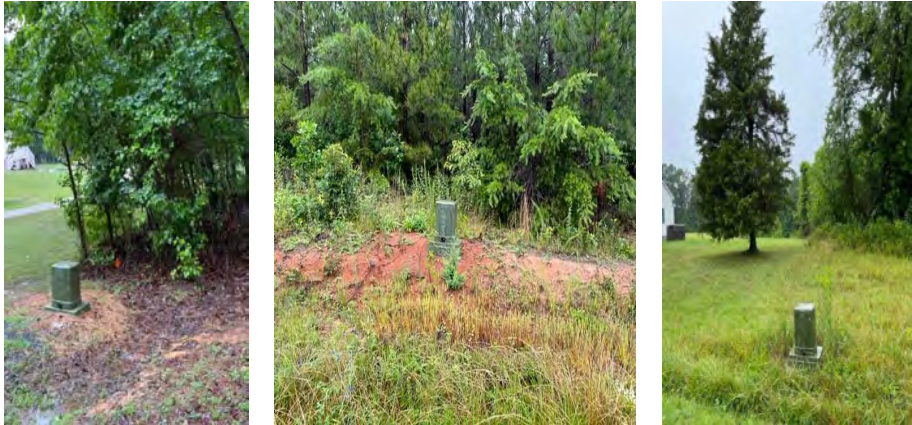
Completed Underground Fiber Installation
